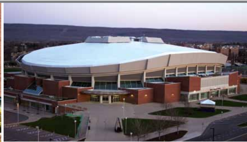
Above: The 16,000 seat Bryce Jordan Center and Medlar Field at Lubrano Park, home of the State College Spikes Single A affiliate of the Pittsburgh Pirates are both next door.
